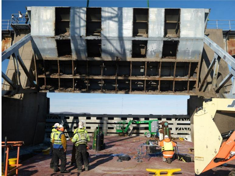
Figure 3 Tainter gate being prepped for testing and removal at Lock and Dam 22
