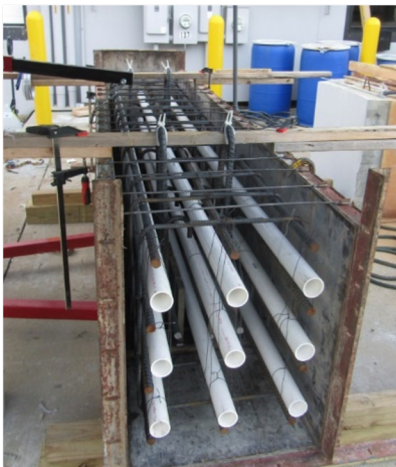
Figure 1: Trunnion beam's rebars and ducts prior to concrete pouring.
