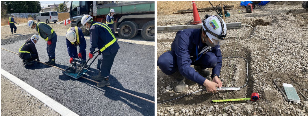
(a) View of construction
