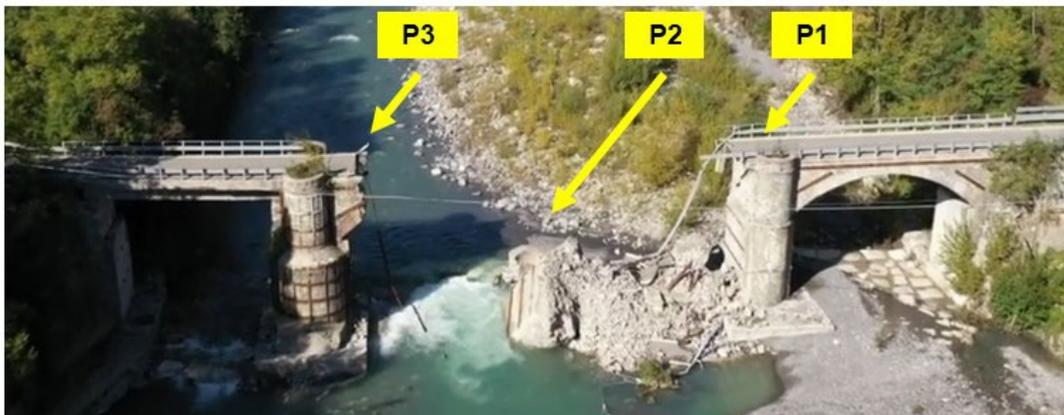
Figure 5: The masonry bridge ruins.
