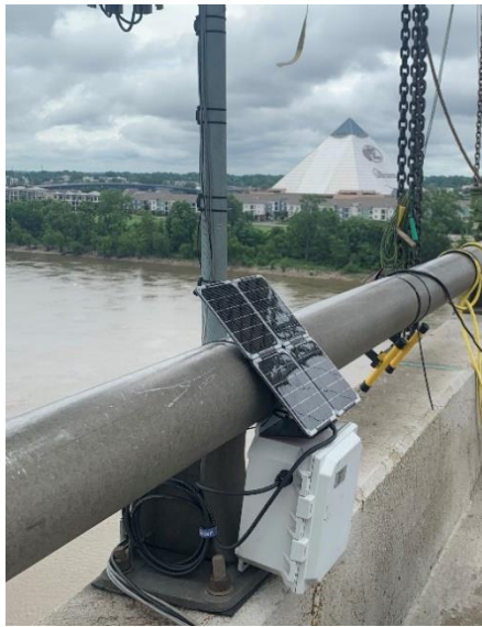
Figure 5. Installed solar powered SeniMax™ gateway on I-40 bridge for data acquisition
