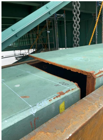
Figure 2. On May 11th, 2021, a crack was detected in main load bearings member of an I-40 bridge in Memphis, Tennessee and as a result, the bridge was closed immediately for the emergency repair.
